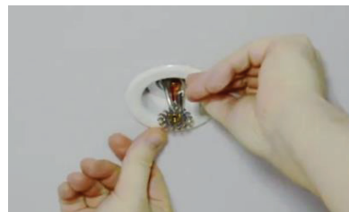
2. Press the escutcheon into place until secured
