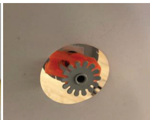
1. Cut holes in the dust ply and fabric diffuser
